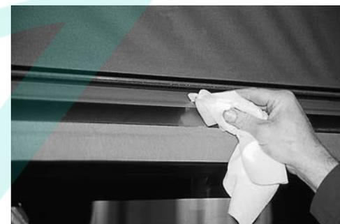
In order to achieve a good sealing, the stripes have to be so thick that the adhesive protrudes a little above and beneath the profile when pushing TOP-RAIL against the surface.
